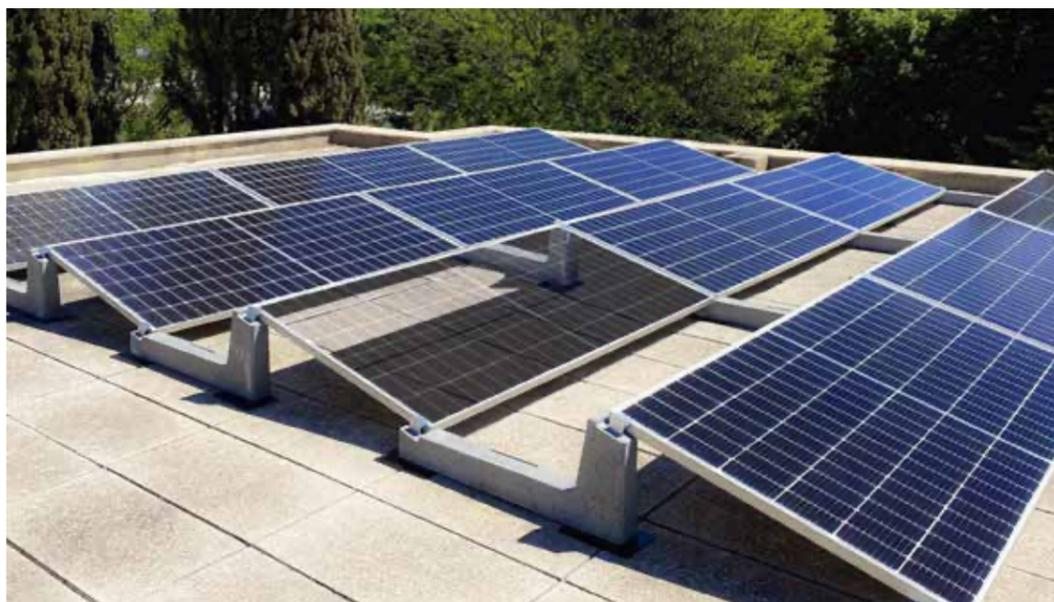
I PRODOTTI DI PUNTA DI SUN BALLAST: A SINISTRA I SISTEMI DI MONTAGGIO CONNECT PER IMPIANTI DI TAGLIA COMMERCIALE E INDUSTRIALE; IN ALTO IL NUOVO SISTEMA NO-FLEX PER IL FISSAGGIO DEI MODULI SOLARI DI GRANDI DIMENSIONI
