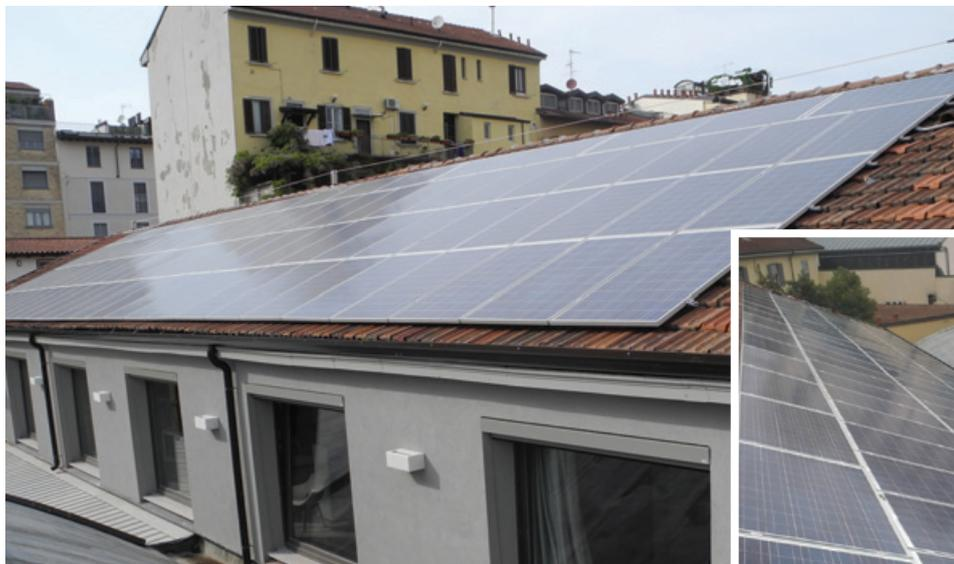
I 90 MODULI SUPER SOLAR PRODUCONO CIRCA 22.000 KWH ALL'ANNO DI ENERGIA PULITA, UTILIZZATA PER IL 70% IN AUTOCONSUMO
